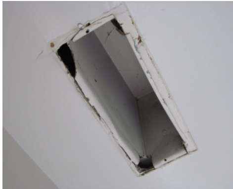
Figure 5. Air sealing opportunity at corners of duct boot where it meets ceiling drywall
