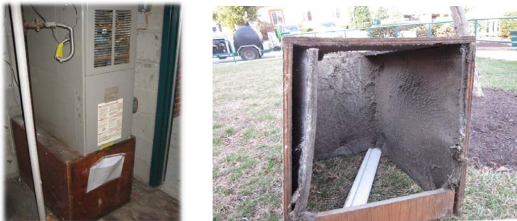
Figure 9. Pre-retrofit furnace and HVAC return plenum
