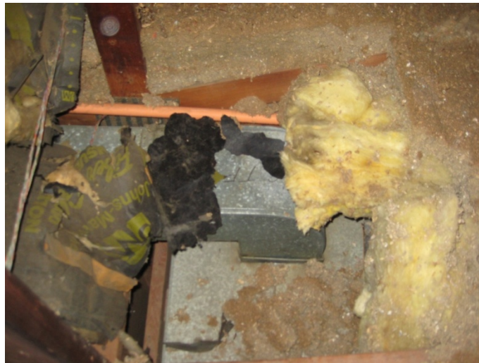
Figure 8. Supply trunk for third-floor apartment exposed to attic (pre-retrofit condition)
