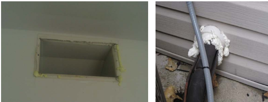
Figure 6. Air sealing of duct register boot and an HVAC penetration
