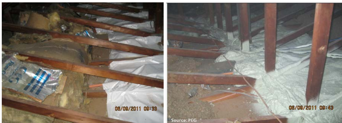
Figure 11. Membrane application followed by SPF application to seal off top of duct bulkhead from attic
