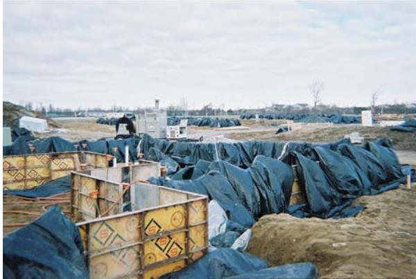
**Figure 5 – Conventional concrete forms**
